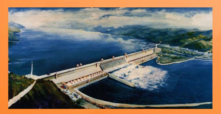
The **Three Gorges Dam** is a <u>hydroelectric gravity dam</u> that spans the yangtaze river by the town of sandouping in yiling district, Yichang, Hubei provience, china. It is the world's largest power station in terms of installed capacity of 22,500 MW.
