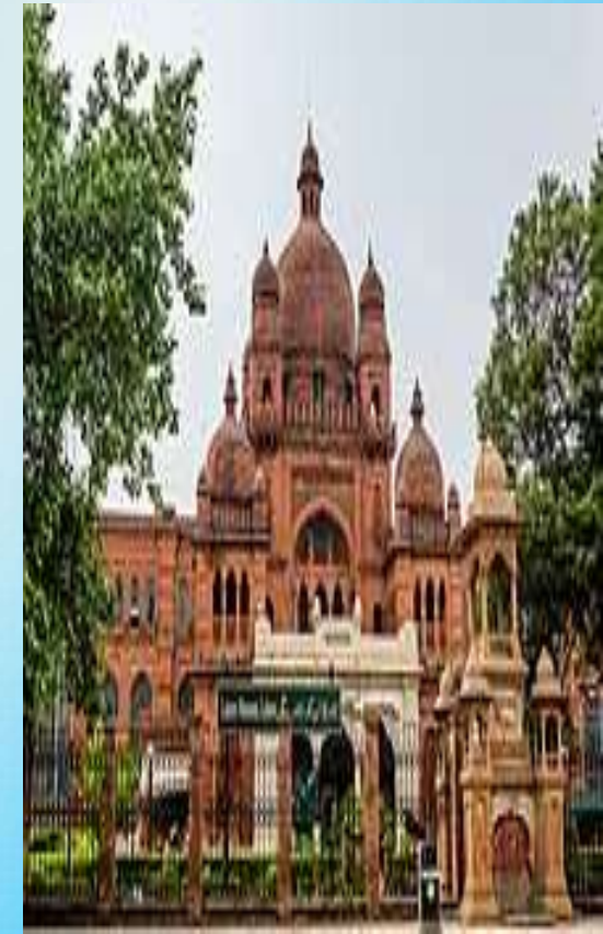
The Lahore Museum building was designed in the Indian Revival architectural style by Sir Ganga Ram.
