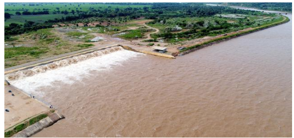
Pattiseema Lift Irrigation scheme
