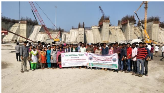
Spillway construction site
