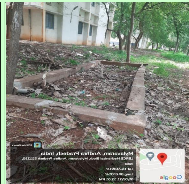
Figure 59: Rain water harvesting pits
