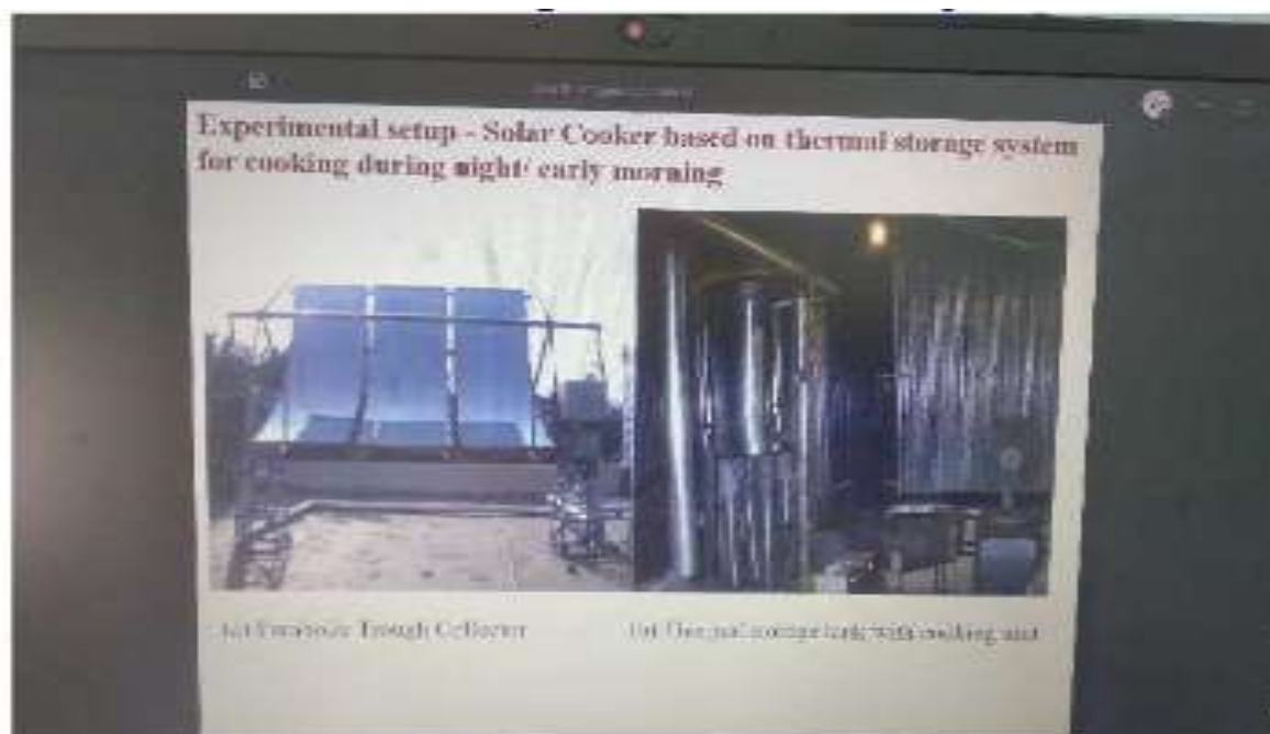
Solar thermal cooker plant at Germany
